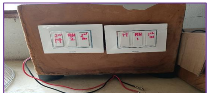
Figure 6 Swapping of Switch for power transmit
