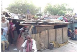
Walls made up of timber & fabric
