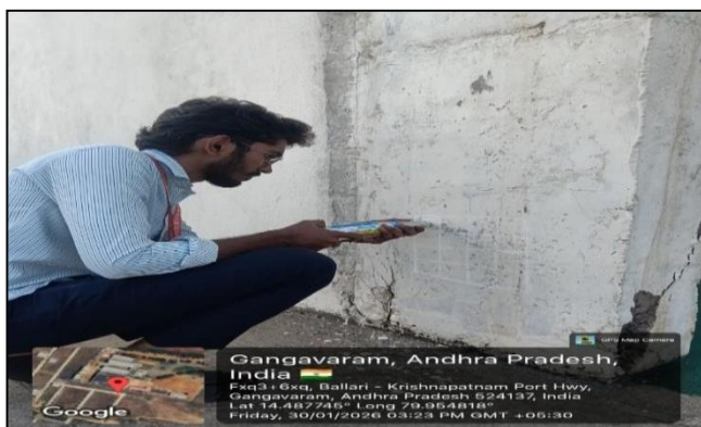
Figure 3 Rebound Hammer Test
