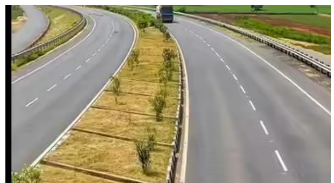
Figure 2 Newly Constructed ‘Plastic Mix’ Roads in Bihar
